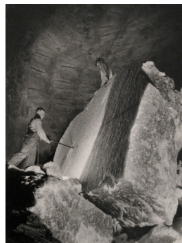
17 Harold Haliday Costain Drilling a 60-ton Rocksalt Block, Avery Island, Louisiana 1934 Chlorobromide Print 14" x 10.75"
