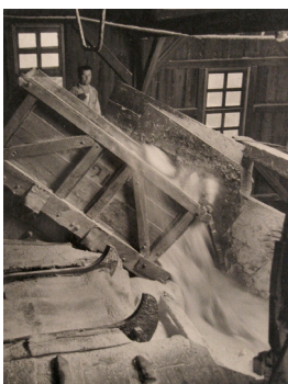
5 Harold Haliday Costain Dumping 3 1/2-ton Rock Salt from the Top of the Breaker into Giant Crusher, Avery Island, Louisiana 1934 Chlorobromide Print 14" x 10.75"
